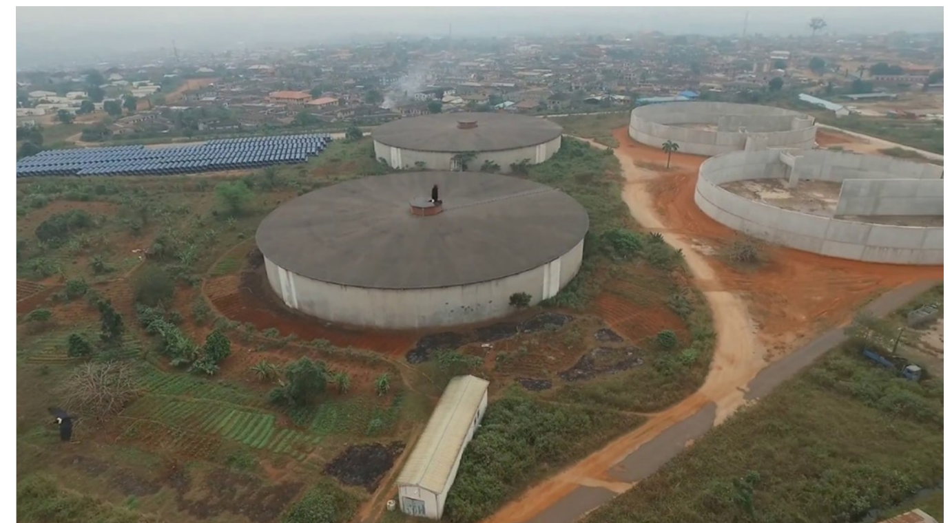
Adiyon Water Treatment Plant, Lagos
